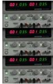
SIX 5 VOLT DC POWER SUPPLIES
